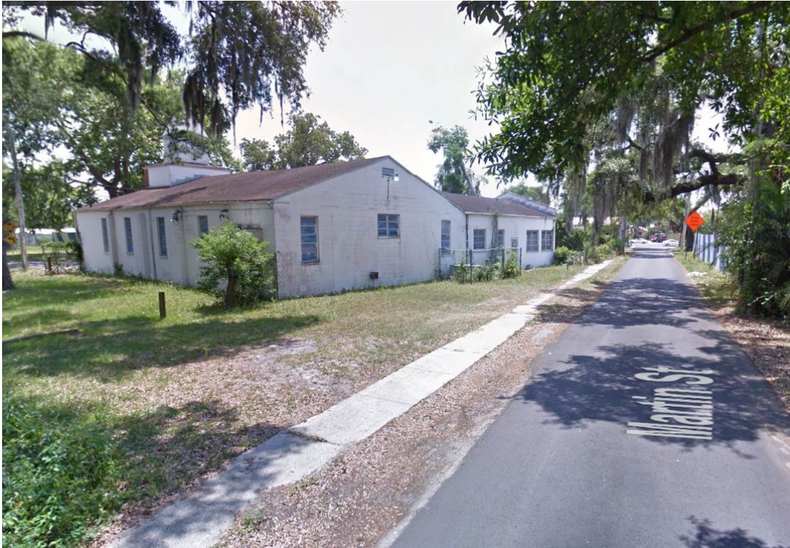
Rear of subject site on Martin Street
